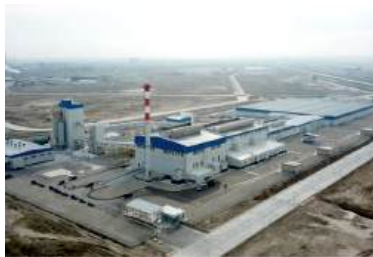
SUMGAYIT CHEMICAL INDUSTRIAL PARK
